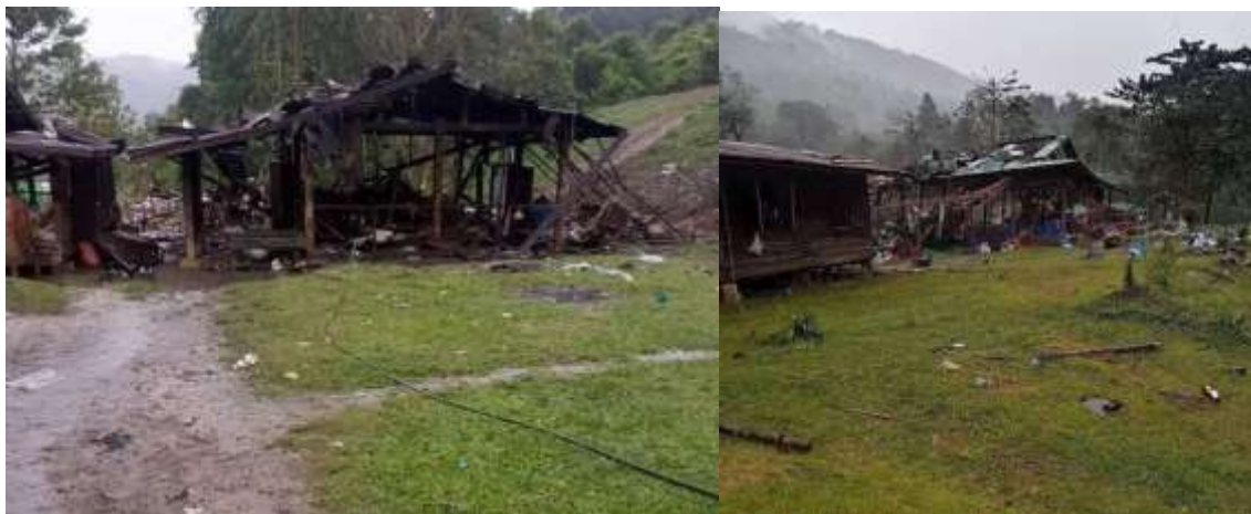
Figure 3: Some structures completely destroyed, located at 25.837176, 96.364021 (Source: Khit Thit Media ).
