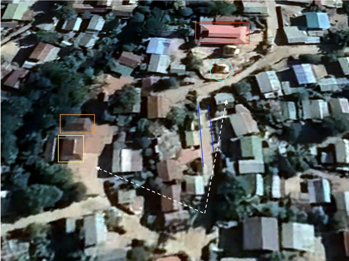
Figure 4: Geolocation of the damages shown in the video footage [22.720263, 95.567659]
